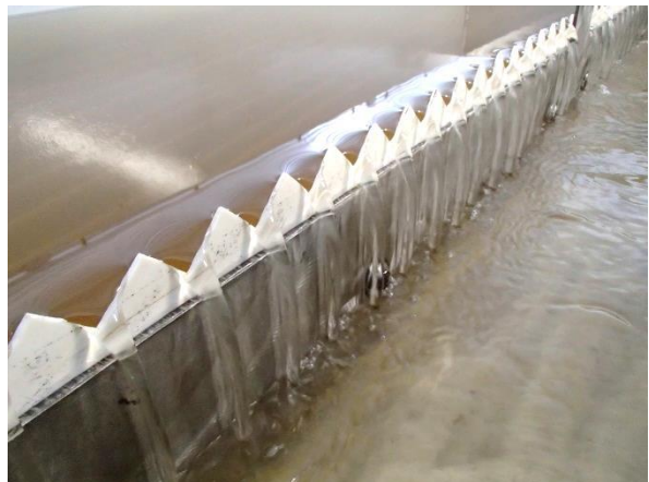
Treated water flowing over the effluent weir
